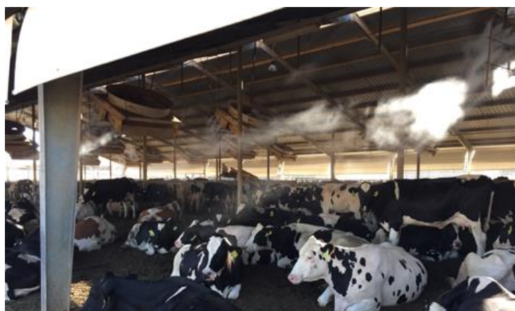
FIGURE 16. HIGH PRESSURE MISTING ATTACHED TO FANS 124 .
