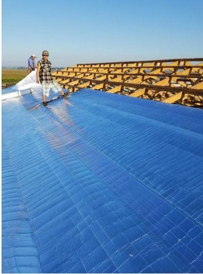
FIGURE 17. INSTALLATION OF RADIANT BARRIER MATERIAL ON A BARN ROOF.
